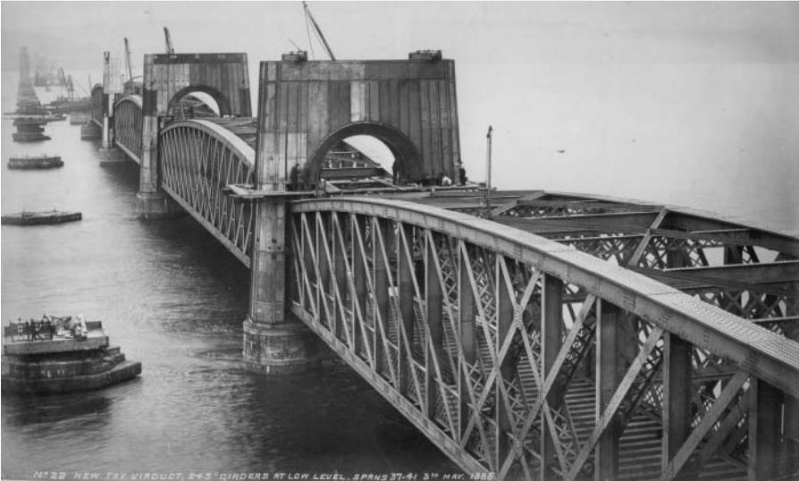
*Photograph showing the new Tay Viaduct during construction, next to the remains of the original viaduct which collapsed during severe gales on 28 December 1879. Photograph dated 3<sup>rd</sup> May 1886.*
