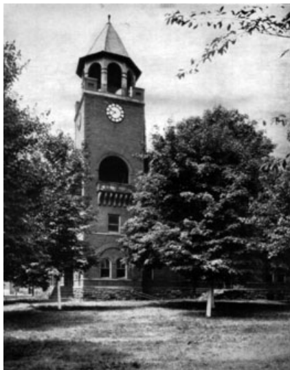
Figure 4. Rhea County courthouse, scene of the action. 1
