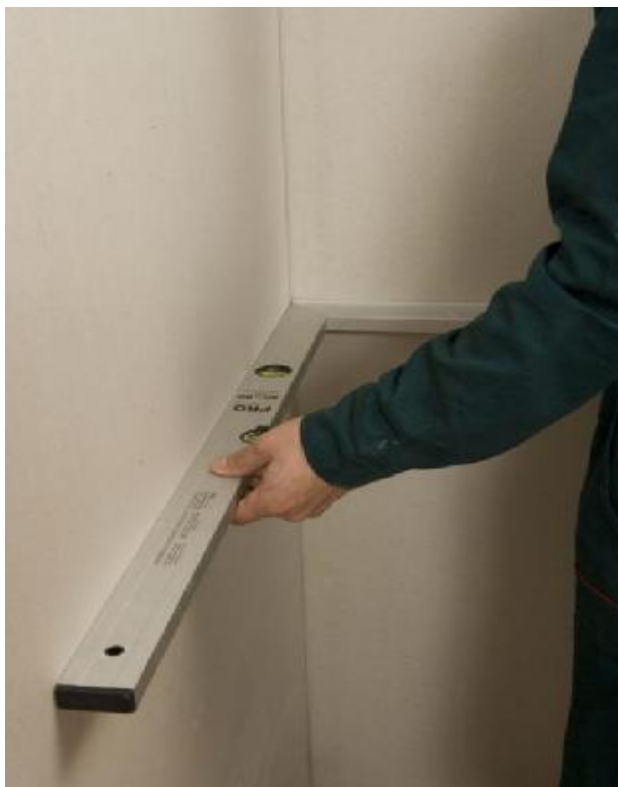
Fig 5. Checking deviation of intersecting planes from the angle specified in the documentation.
